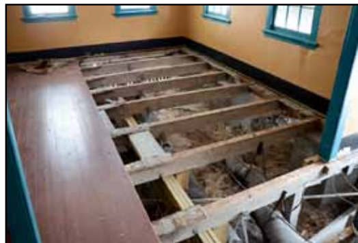
Flooring removed in a section of the parlor.
